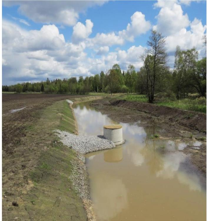
Fig 3. **"Classical"** IBZ. At least 10 m wide with a 4 m wide drivable infiltration bank. Incoming drainpipes are separately emptied in the collecting ditch. They are usually temporally flooded during rainy weather conditions.
